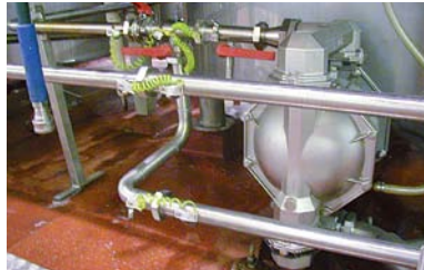
3" sanitary pump used to transfer cosmetic basis for shampoos
