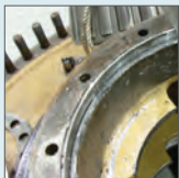
Pitting on bearing
